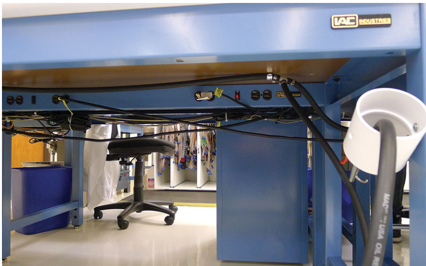
To clean up the previous spaghetti mess of electrical wires, Cicoil mounted an electrical channel to the rear cross-member of each workbench. Photo courtesy IAC Industries Inc.
